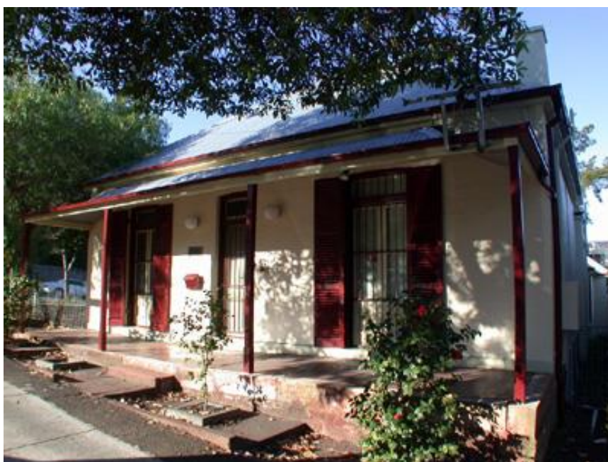
Figure 16 - 52 Sorrell Street opposite the subject site
