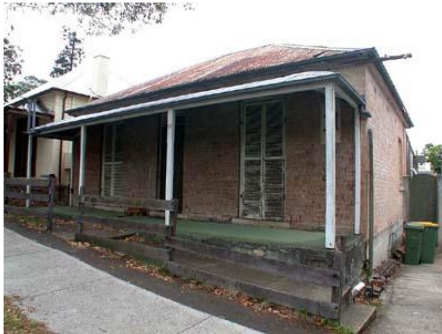
Figure 15 - 50 Sorrell Street opposite the subject site
